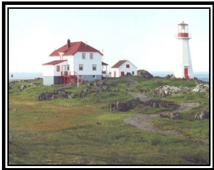
Cape Bauld - Lightkeeper's Residence
